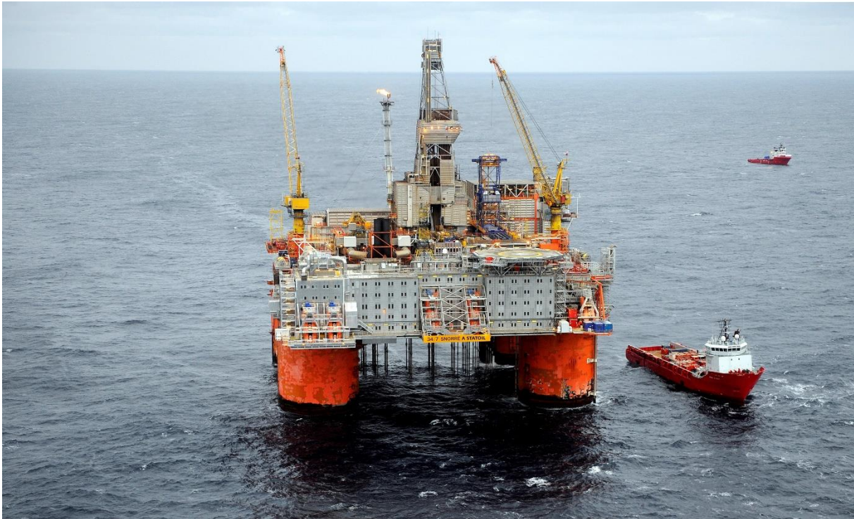
Figure 5: The integrated production, drilling and quarters unit Snorre A in the Norwegian North Sea. Photo by: Harald Pettersen
